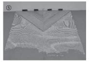
Apply adhesive with the Hamberger special spreader D along the chalk line laid out in the centre. The width of the adhesive application equals the width of a covered width to the left and the right of the chalk line. Lay the boards previously laid out and fitted together into the glue layer. Only apply adhesive for the area you can install in 15 minutes. (Total amount of adhesive applied depending on the quality of the substrate 800–1000 g pro m²)
